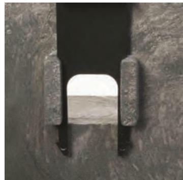
Winterized Cable Drop Side
